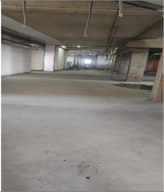
M.O.T Flooring Complete
