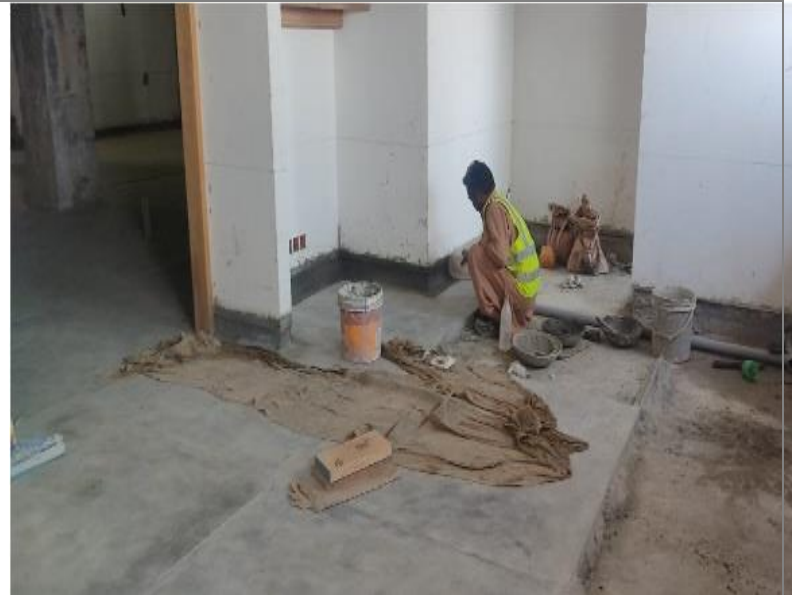
Flooring and Skirting Work of Holding Area in Progress
