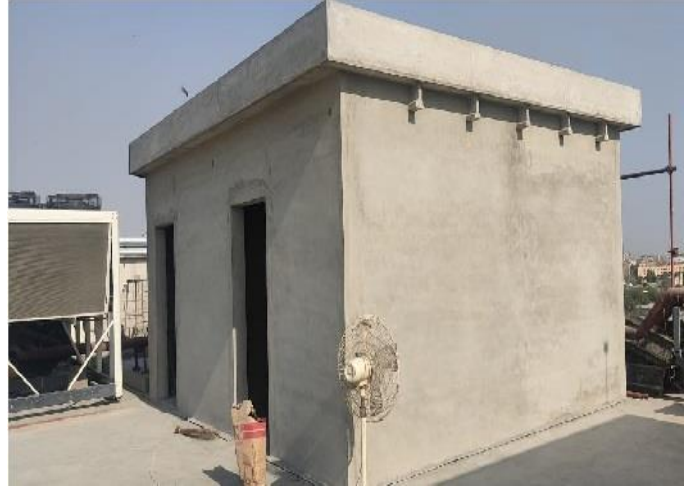
LV and Pump Room Finishing Work
