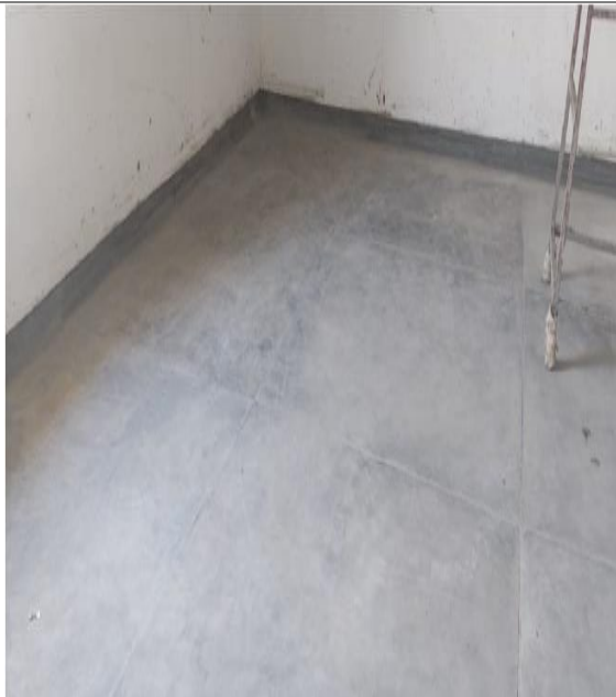
Non Sterile Supply Room Flooring Complete
