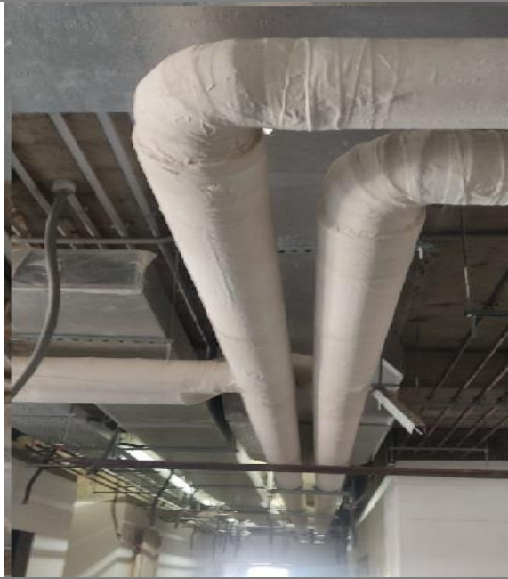
Chilled Water Pipe Insulation
